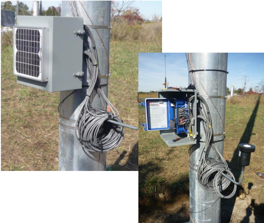
○ 50 m meteorological tower
